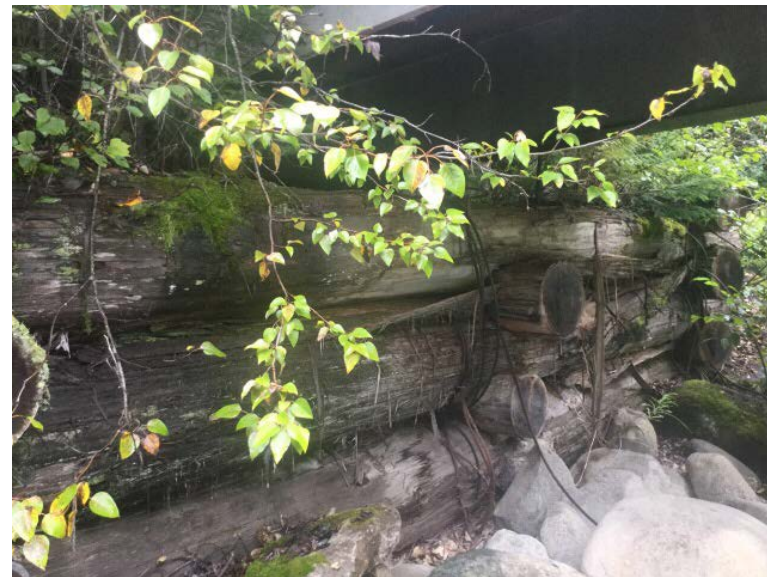
Right Bank Abutment when facing downstream
